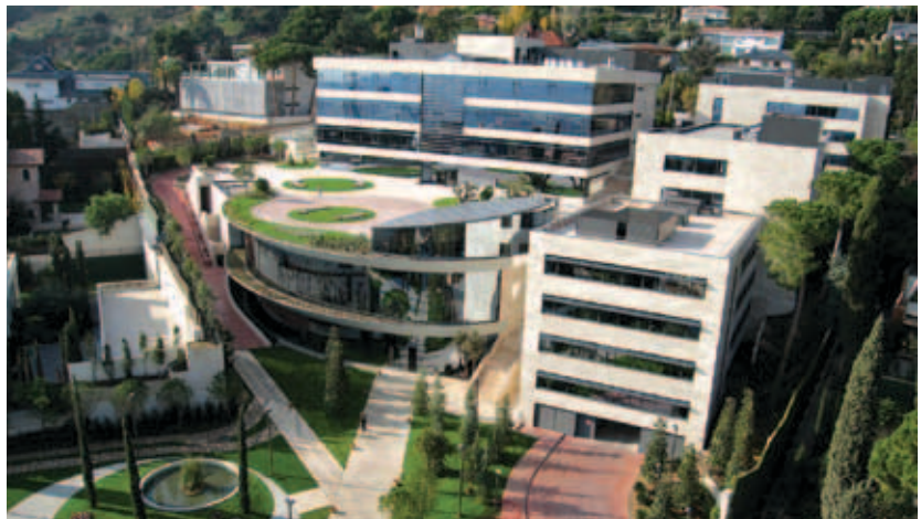
View of IESE’s Barcelona campus.
