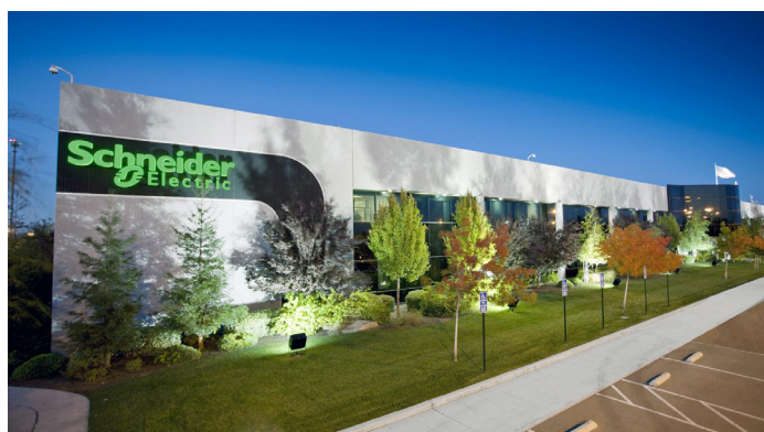
Figure 1. Schneider Electric’s Innovation Center in Silicon Valley
