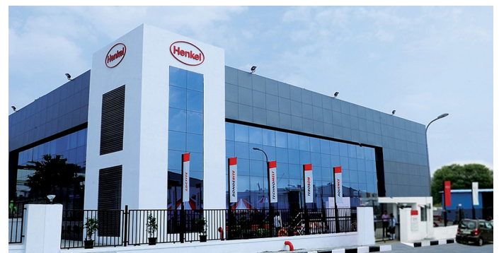
Figure 4. Henkel’s Innovation Center in Pune
