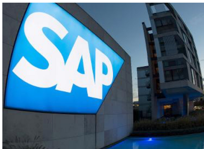
Figure 11. SAP headquarters in Walldorf
